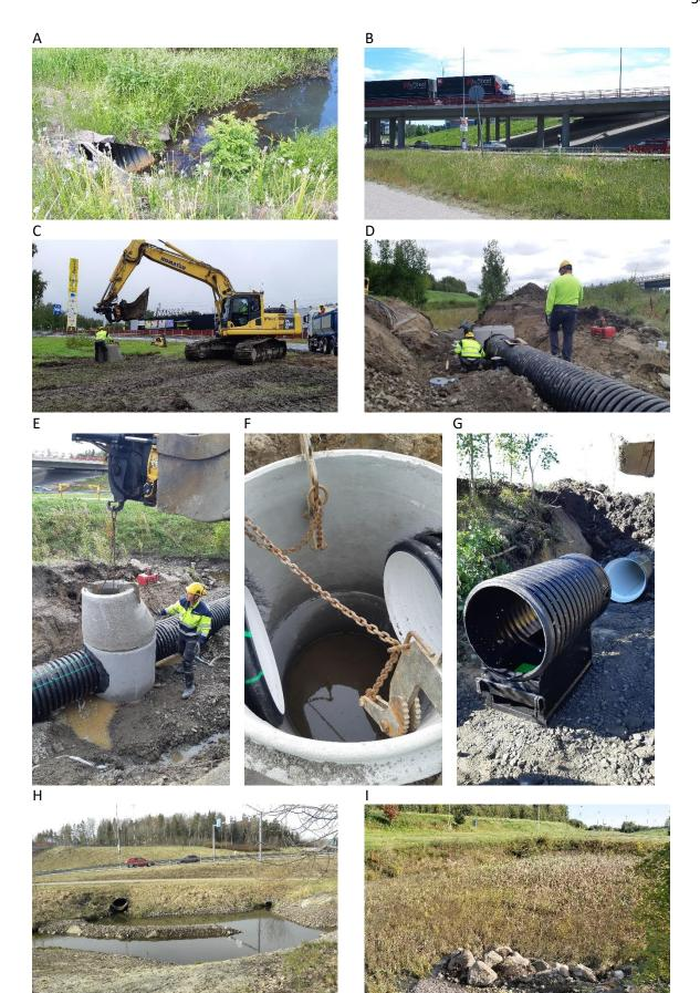
Figure 47 Highway 6 ramp CW and construction: A...B) CW before implementation, C...G) construction, and H... I) CW site after modification. H) influent to settlement pond before the filter, I) secondary settlement pond and outflow pipes from filter.
