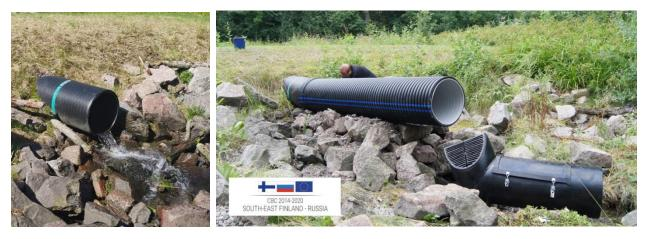
*Figure 44 Outlet pipe from 1<sup>st</sup> basin before and after the filter installation.*
