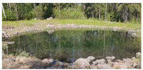
Basin 1: influent from drainage system (2019). Water quality was monitored as taking a composite sample. Settling tank in drainage system is located near influent pipe.
