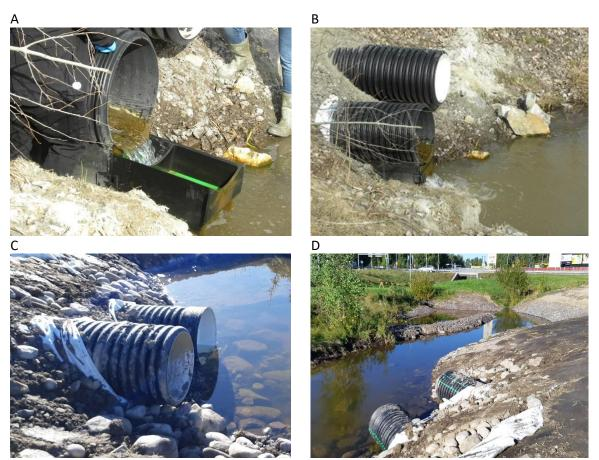
Figure 48 Highway 6 ramp CW: A and B) Outflow EM-shungite filter installed at the end of the black pipe. The upper "white pipe" is backup pipe for flood water. C and D) influent from the small upper pond to the filter.
