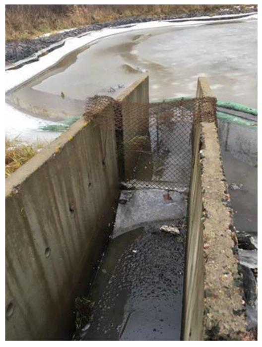
Figure 57 Supply ditch with grate and oil booms
