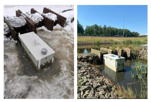
Figure 100 Installation of filter in the stormwater retention pond.
