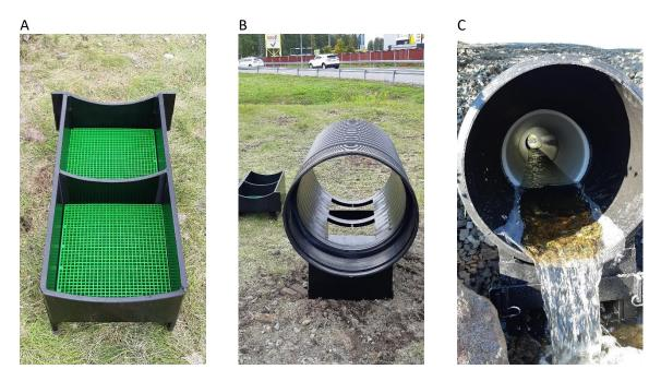
*Figure 37 Horizontal flow filter implements at ramp of highway 6 site: A) sledge for filter media, B) pipe unit above the sledge, C) flow out from the pipe unit. Horizontal water flow pass grid above the materials and flows partially through the filter materials.*
