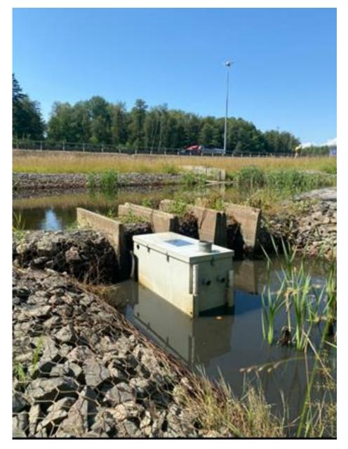
Figure 58 The main retention pond and outlet with final filter.
